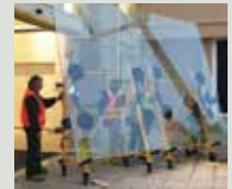
Lifting Capacity Upgrade
